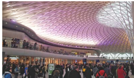
VINCI PLC's £180m redevelopment of the King's Cross Western Range building and the extension of the Western Concourse completed without any loss of service.
