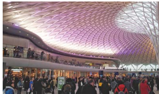
VINCI PLC's £180m redevelopment of the King's Cross Western Range building and the extension of the Western Concourse completed without any loss of service.
